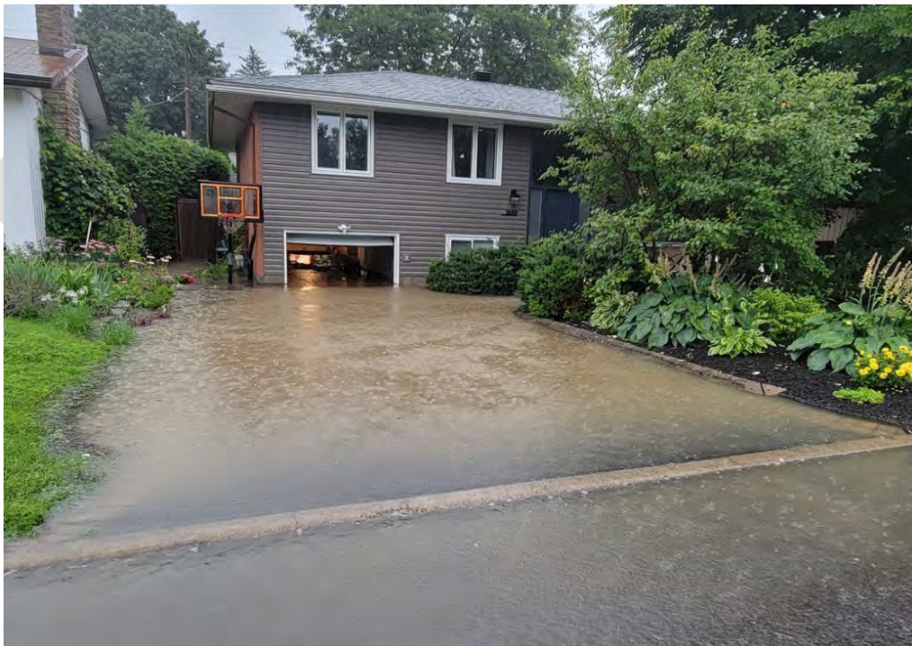
Figure 8 – Flood on Colman Street
