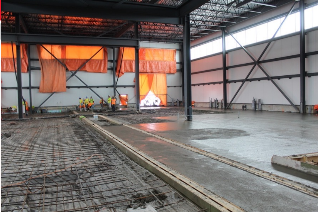
Concrete slab flooring being poured
