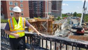
The first high wall is complete. Formwork, rebar and concrete placement for wall construction continues. Work on the stair tower is expected to begin soon.
